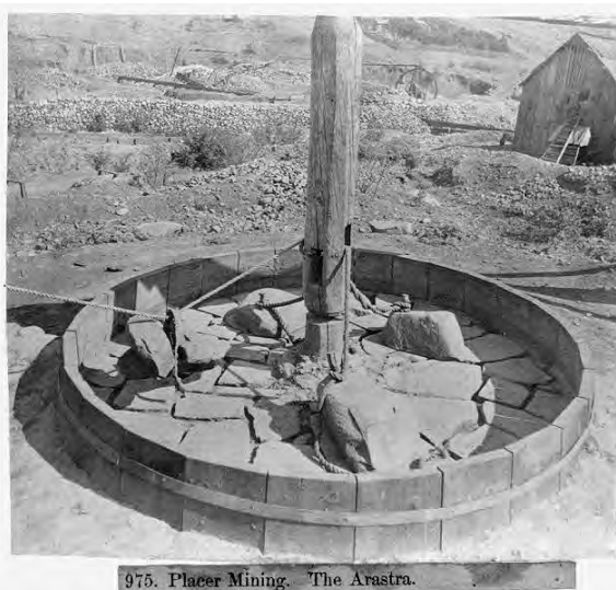
Placer Mining: The Arrastra (Lawrence & Houseworth, 1866)
