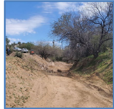
Lake Pleasant – Agua Fria – graded and repaired road and wash area.
